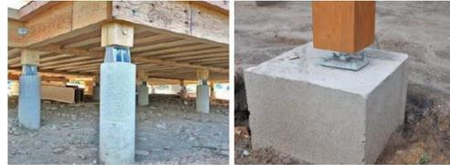
OPTION D'INSTALLATION: PLATEFORME MONTÉE SUR PILOTIS MASSIF EN BÉTON
